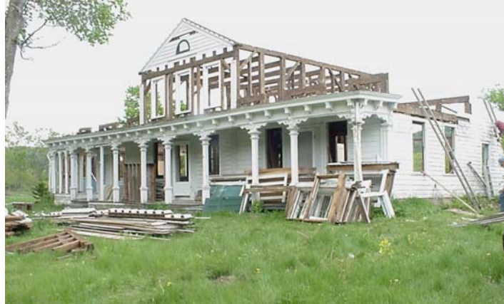
Dismantling of Bruchmann residence, May 2000
